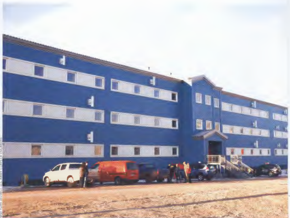
The 54 person dormitory under construction.
