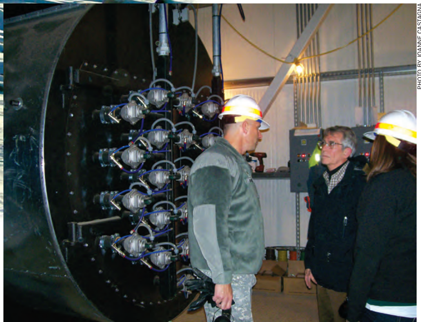
New York District Commander Col. John R. Boulé explains the workings of one of several exhaust-gas boilers the Army Corps built at Thule Air Base.
