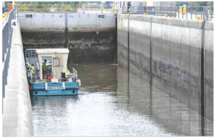
A vessel traveling through the Troy Lock and Dam. photo: Michael Embrich, Public Affairs, New York District, USACE
