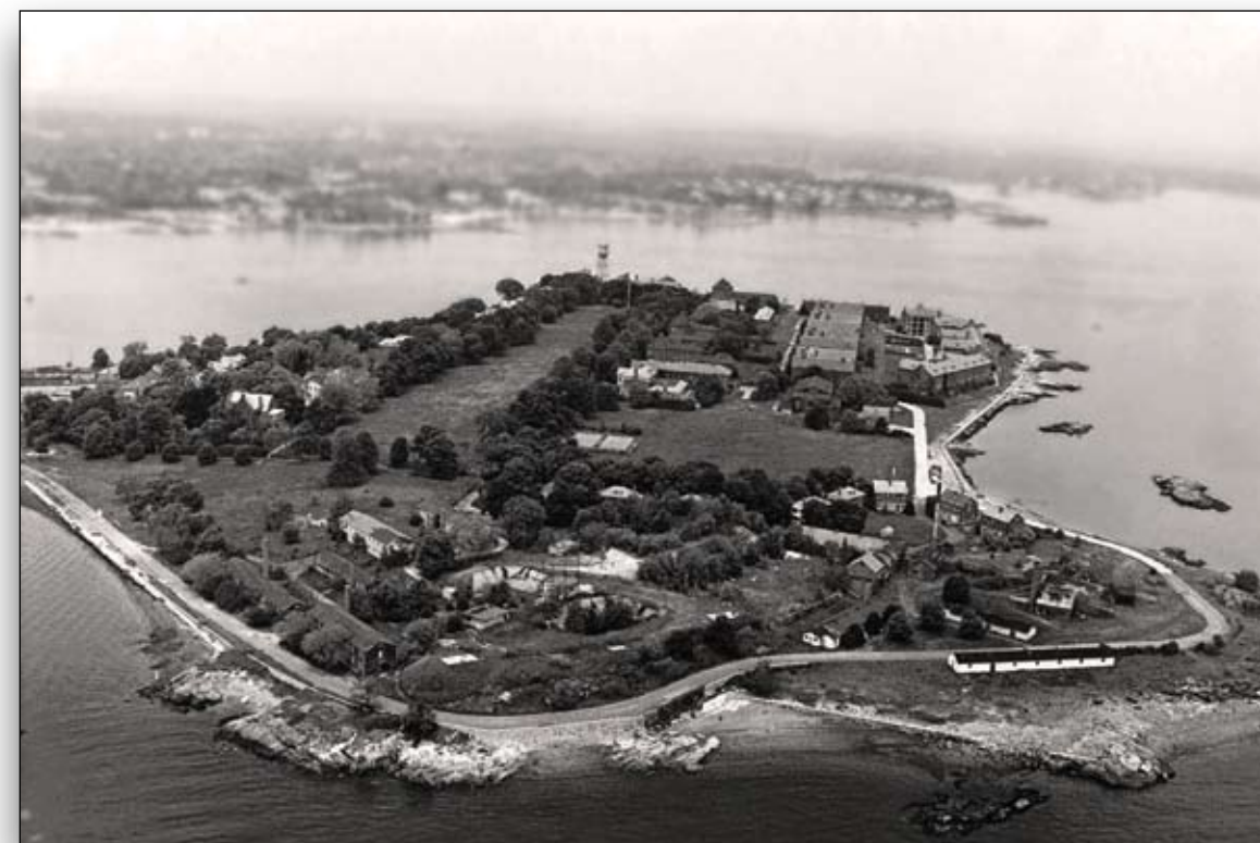
TOP: Oblique aerial photograph of Fort Slocum, taken November 15, 1961. The fort's last military incarnation was during that time when it served as a missile command base. Since then, the island has laid dormant and the public has been denied access. (Photo from Fort Slocum Alumni and Friends Collection, Michael J. Cavanaugh, Los Angeles, CA, custodian.) TITLE PAGE: Fort Slocum Post Headquarters, built in 1909. (Photo by Tetra Tech EC, Inc.)
