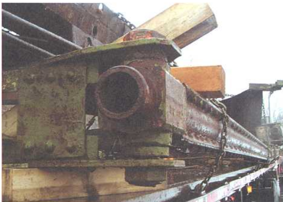
Figure 2: One of the Phoenix Columns is visible on the truck during moving day.
