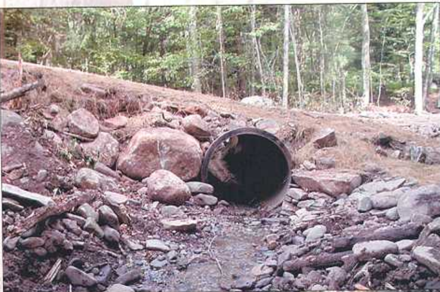
Culverts channel streams and water runoff to filtered areas. Road is crowned and trenched.
