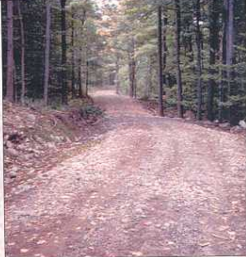
Culverts channel streams and water runoff to filtered areas. Road is crowned and trenched.
