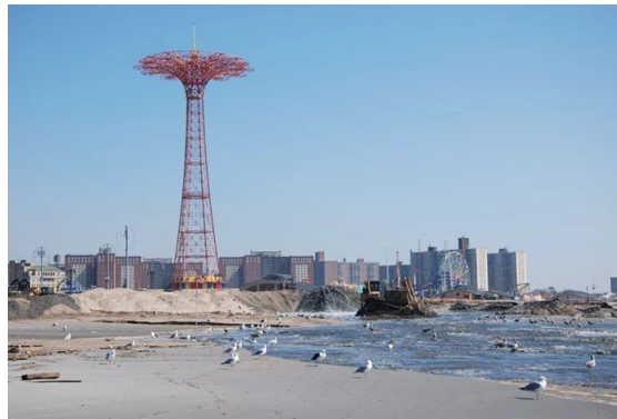
Sand being pumped onto Coney Island Beach, New York. Credit: Public Affairs, New York District.
