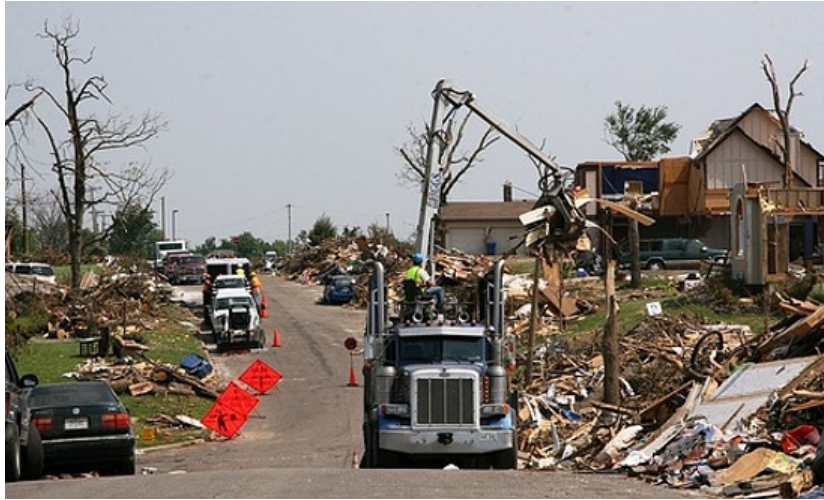
Trucks removing the estimated 3 million cubic yards of debris left by the tornado. Image courtesy of U.S. Army Corps of Engineers and John Daves.
