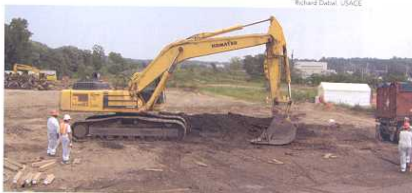
Above: Contractors supervise an excavator loading radioactive soil for off-site removal and disposal.
