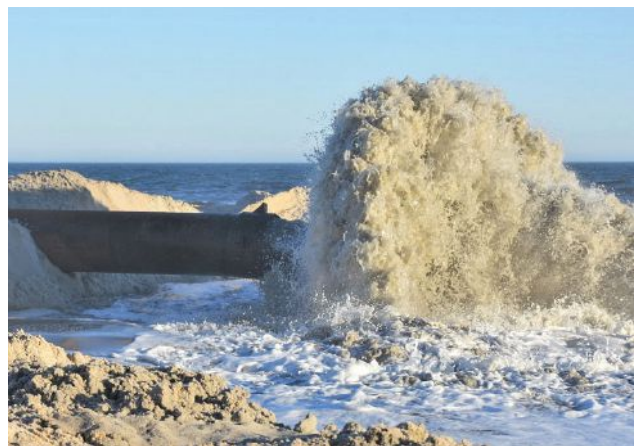
Sand replenishment pumps sand through pipelines onto several beaches in order to prevent elevated ocean waters from flooding coastal communities.
