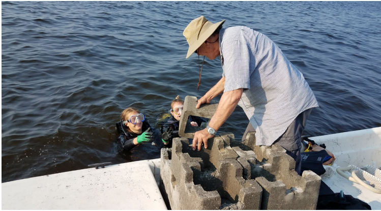
NY/NJ Baykeeper divers in the Raritan Bay being handed an oyster castle, a concrete block, that will be stacked to make a pyramid to provide habitat structure for the oyster reef and other marine life. Photo: NY/NJ Baykeeper.
