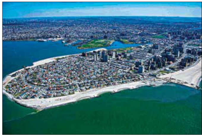
Aerial image of the Sea Gate portion of the Coney Island peninsula showing the completed T-groins in 2016. Credit: USACE.
