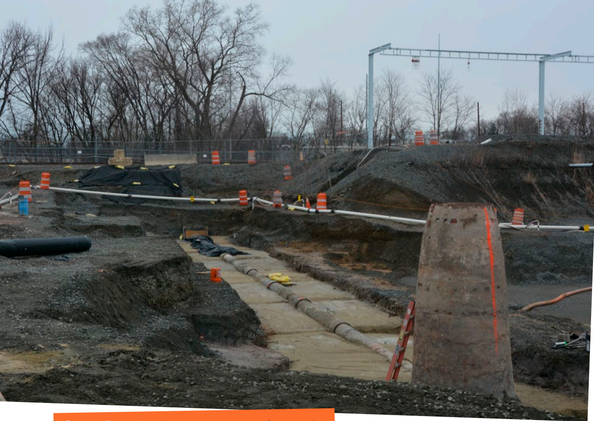
Contaminated soil is removed from the Maywood site. (Photo: Nayelli Guerrero/USACE)
