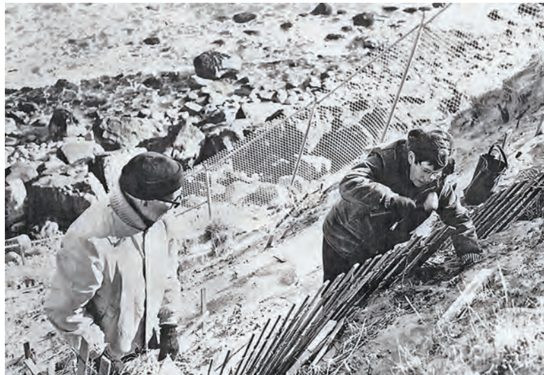
Giorgina Reid using her reed terracing method to stabilize the Montauk Point Lighthouse cliffs in the 1970s. (Photo courtesy of Dan's Paper)
